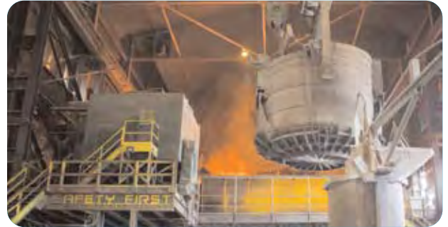
Nucor Steel optimized its steel melting process to drastically reduce electricity consumption.
